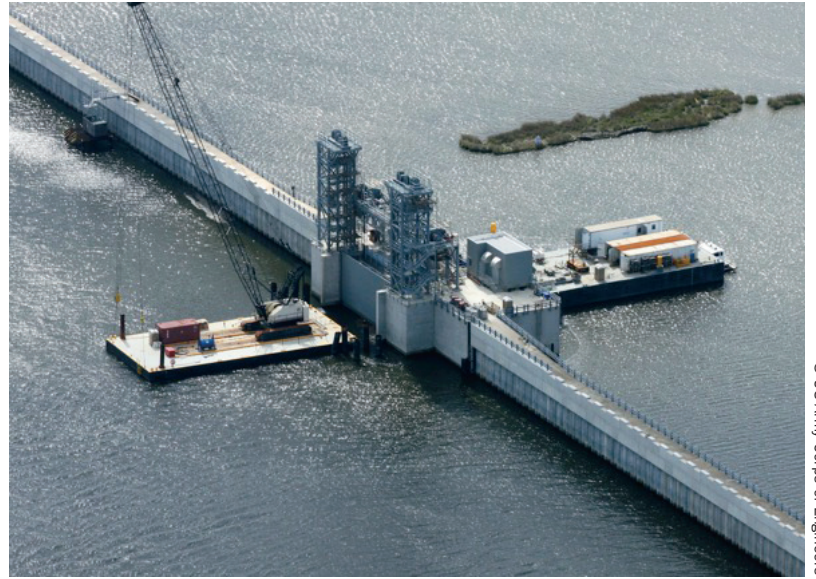
Example of vertical lift gate.
